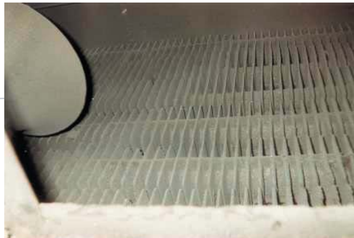
ECONOMIZER sections after one months process with SONIC CLEANING
