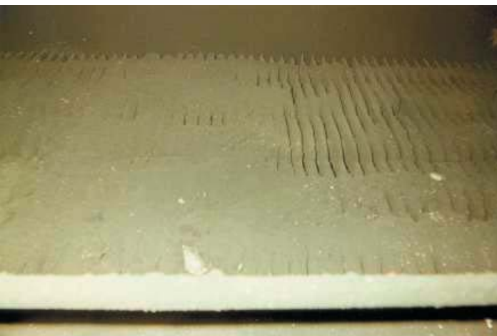
ECONOMIZER sections after one months process without SONIC CLEANING
